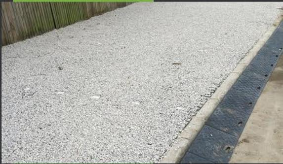
**1.** Install edge retention as specified: Either tantalised timber boards, concrete, steel or plastic kerbs as appropriate
